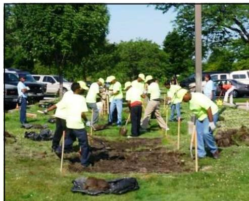
A bioswale is a shallow depression designed to store and convey storm water runoff toward a discharge point, in this case a storm drain. This bioswale will collect water from the surrounding marina parking lot. Roughly 900 non-invasive perennial plants and 28 cubic yards of amended soil will slow down the storm water, promote infiltration and remove contaminants before they reach Euclid Creek and Lake Erie. The storm water is expected to move through the system in less than 48 hours.
